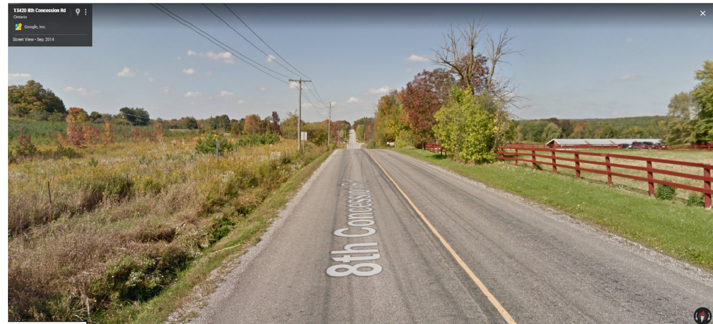
VIEW ALONG 8TH CONCESSION LOOKING NORTH AT APPROX. STATION. 2+860
