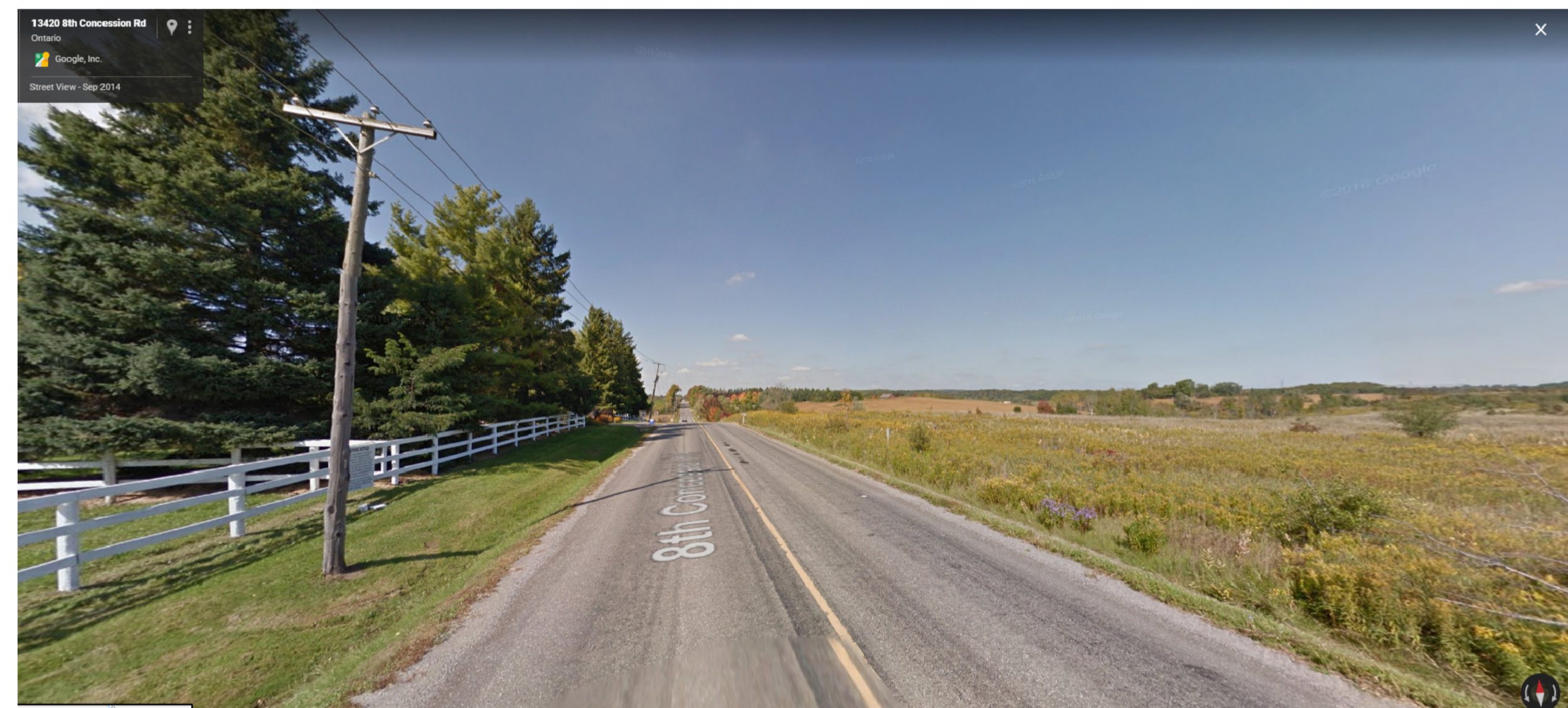
VIEW ALONG 8TH CONCESSION LOOKING NORTH AT APPROX. STATION 2+100
